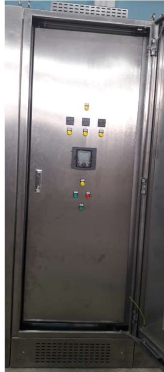
PANEL POMPA 3 x 200KW
